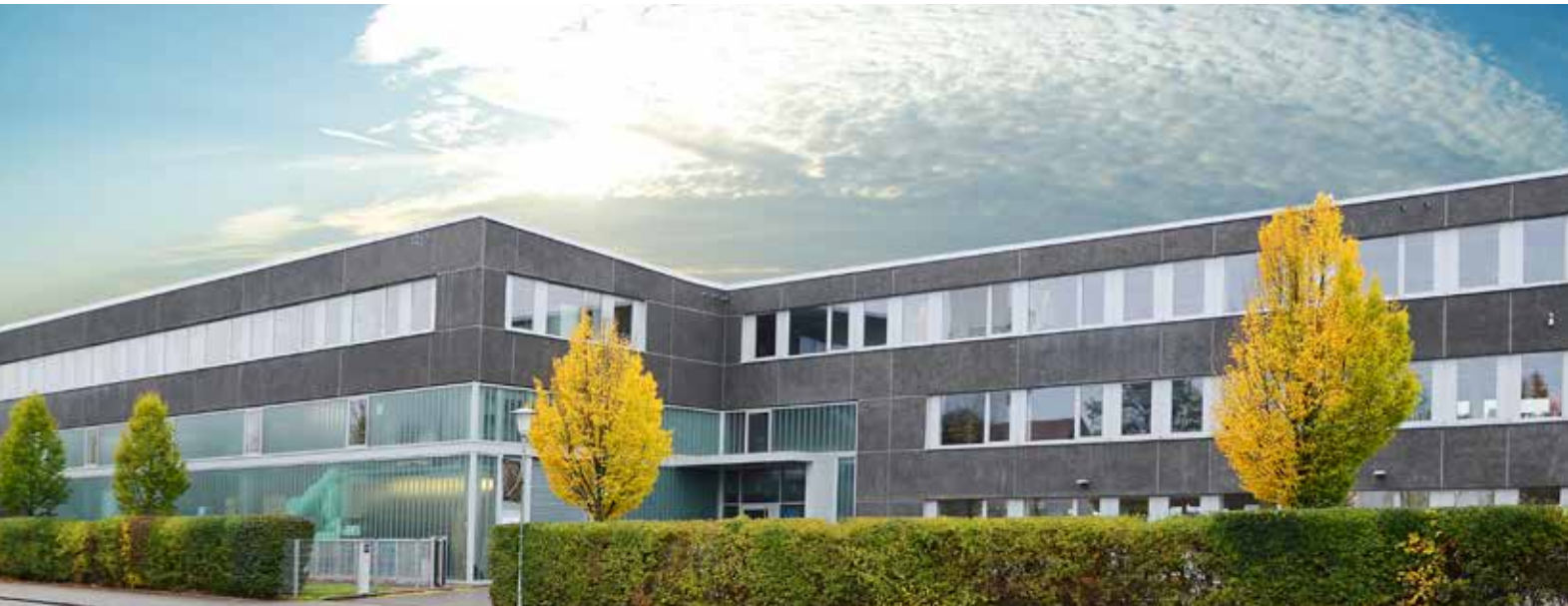
Distec Headquarter in Germering near Munich
